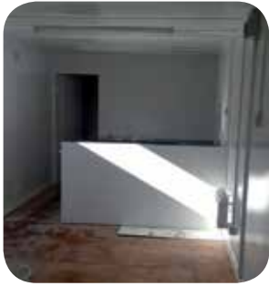
The Community Hub in renovation stage
