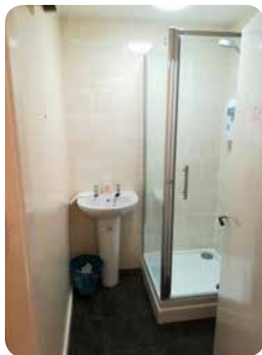
New bathroom in the community flat
