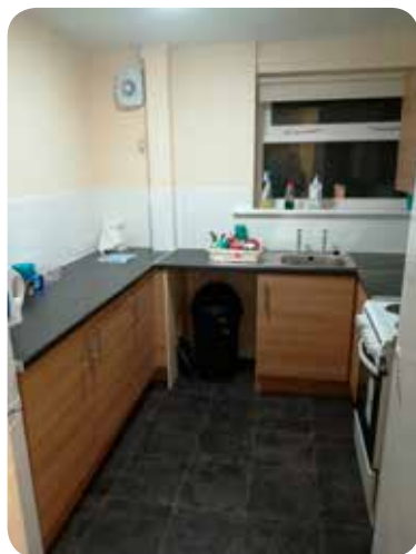
New kitchen in the community flat
