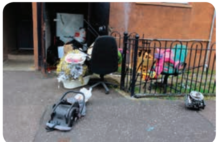
An example of an overflowing bin store at Hailesland
